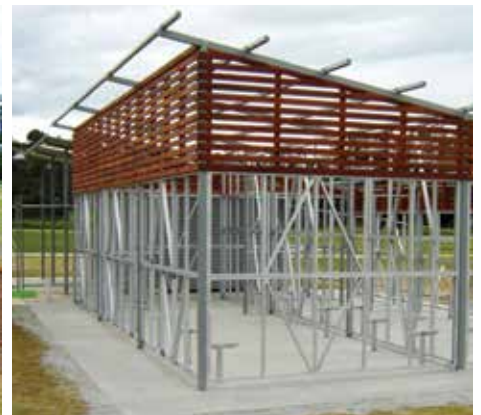
STEEL FRAMEWORK AND WALLS ON-SLAB
