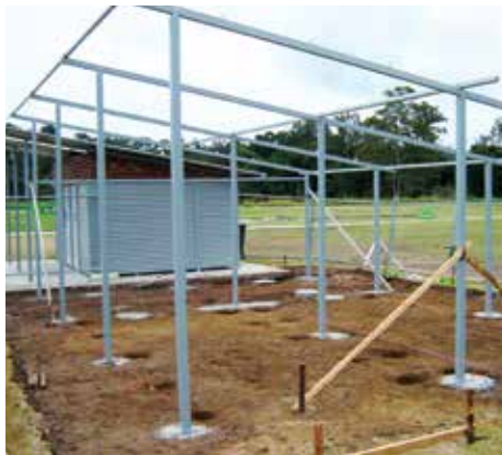
STEEL FRAMEWORK WITH FOOTINGS
