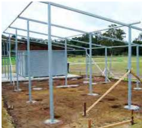
STEEL FRAMEWORK WITH FOOTINGS
