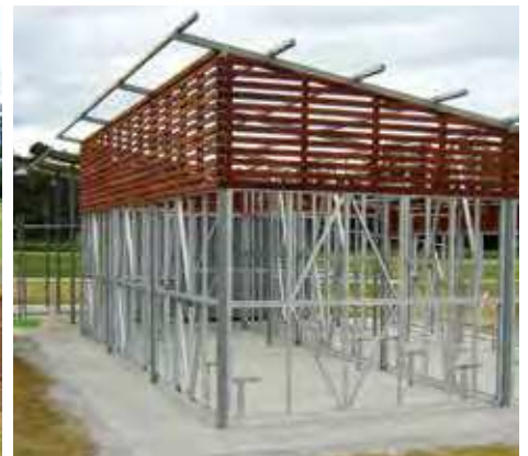
STEEL FRAMEWORK AND WALLS ON-SLAB
