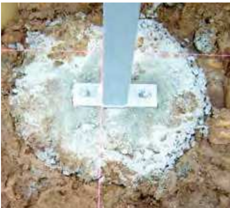
STEEL BOLT-BELOW SLAB FOOTING
